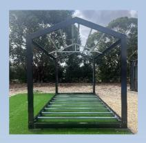
18. Use the **Self-Drilling Screws** and screw them into the plates sticking out of the Triangular Roof Central Support Beam and the C Channel Roof Support Beams.
