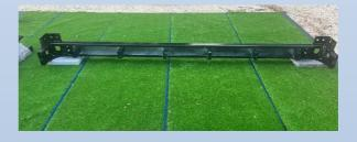
4. Get the **Bottom Long Beam** and place it in-between the 2 Corner Support Pieces that are 6 meters apart. Slide the bottom long beams into the Corner Support Pieces and then secure it by using the small bolts with nuts.
