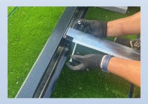
8. With the drill go around to each bolt and nut and tighten it to secure it. You will have a complete base with floor support now.
