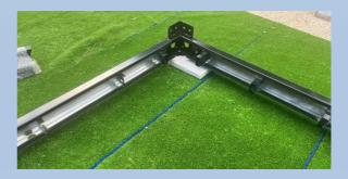
5. Repeat step 3 to the opposite side. With the drill go around to each bolt and nut and tighten it to secure the base
