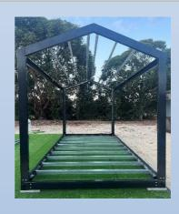
17. Place the **Triangular Roof Central**Support Beam in the centre of the Roof Straight beams. Use the Small Bolts and nuts to secure the triangular roof central support beam to the plate that is in the centre of the Roof Straight Beam.
