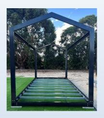
15. Get **the C Channel Roof Support Beams** and put them between the Roof V Shaped Beam. They C channel will slide into the black brackets that are coming out of the Roof V Shaped Beam. Secure them with **the Medium Bolts** and nuts.
