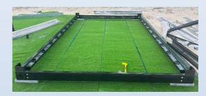
7. Then get the **Square Floor Support Tubes** and insert them into the black brackets that are coming out of the Bottom Long Beam. Then get the **Long Bolts** with nuts and place them through the black beam and square tube to secure it.
