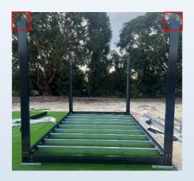
11. Place the **Roof V Shaped Beam** between the 2 Corner Arms which are approx. 3m apart. Secure these with the **Small Bolts** and nuts. Repeat this to the other side.
