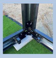
10. Ensure the lower part of the slant corner arm is facing out.
