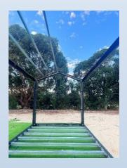
16. Repeat the above until all 6 Channel Roof supports are in. Use the drill to tighten the bolts.
