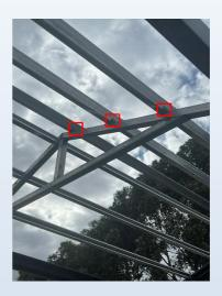
19. Lastly place the Wall Support Beams in the centre of the Bottom Long Beam and the Roof Straight Beam. Use the Self Drilling Screws to screw the Wall Support Beam in
