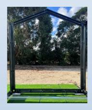
12. Place the **Roof Straight Beam**between the 2 Corner Arms which are approx. 6m apart. Secure these with the **Small Bolts** and nuts. Repeat this to the other side.
